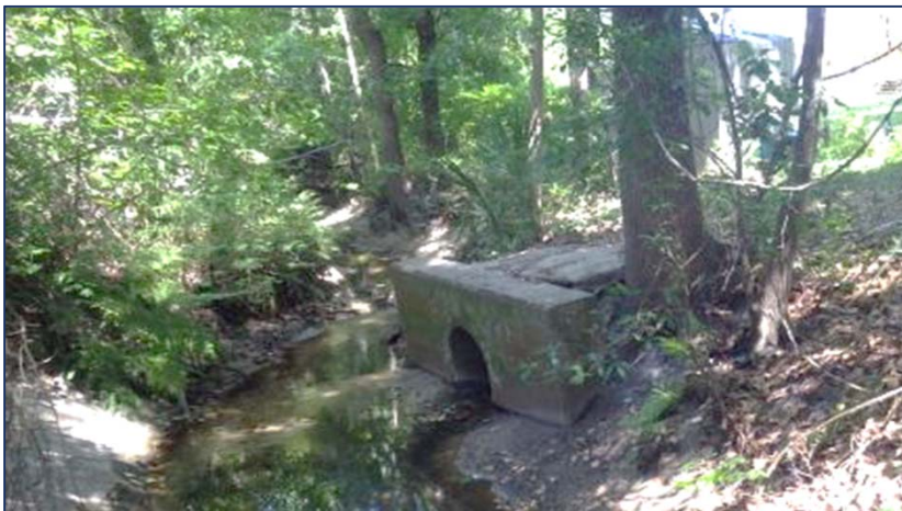
Major Outfall, City of Jacksonville Public Works
