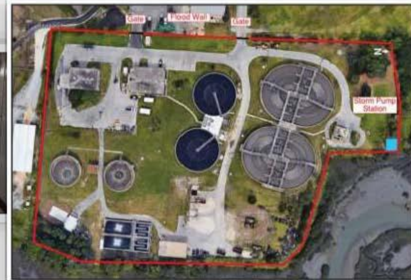
Figure 10: Perimeter Flood Wall and Pump Station
