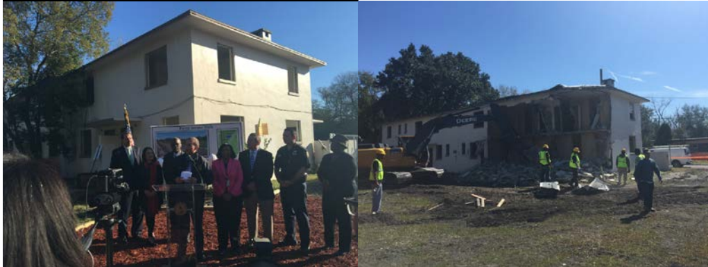
Payne Avenue Walk Groundbreaking and Demolition
