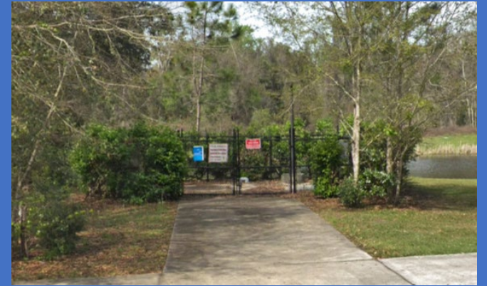
McGrits Creek Park / Low Brantley Pump Station
