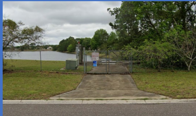
Sandalwood Canal Pump Station
