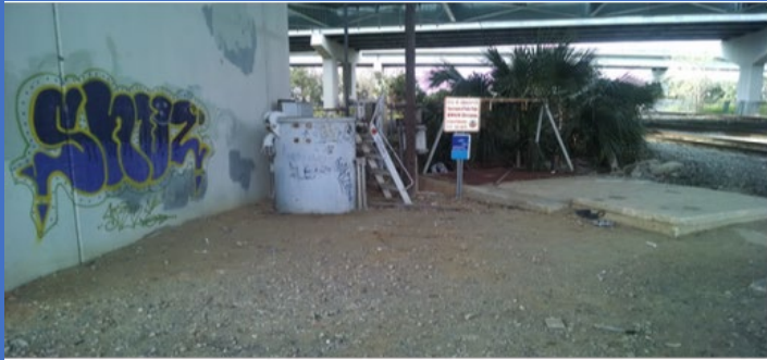
Myrtle Ave Pump Station
