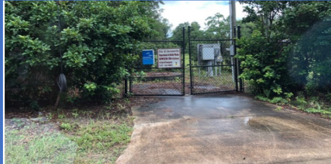
Bradley Road Pump Station
