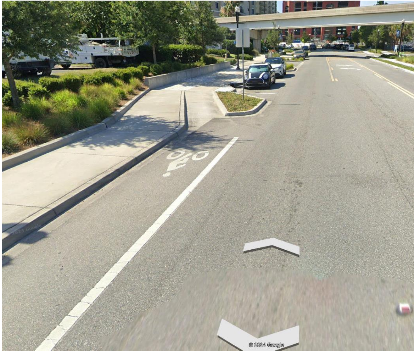
Existing facilities along Riverplace Blvd
