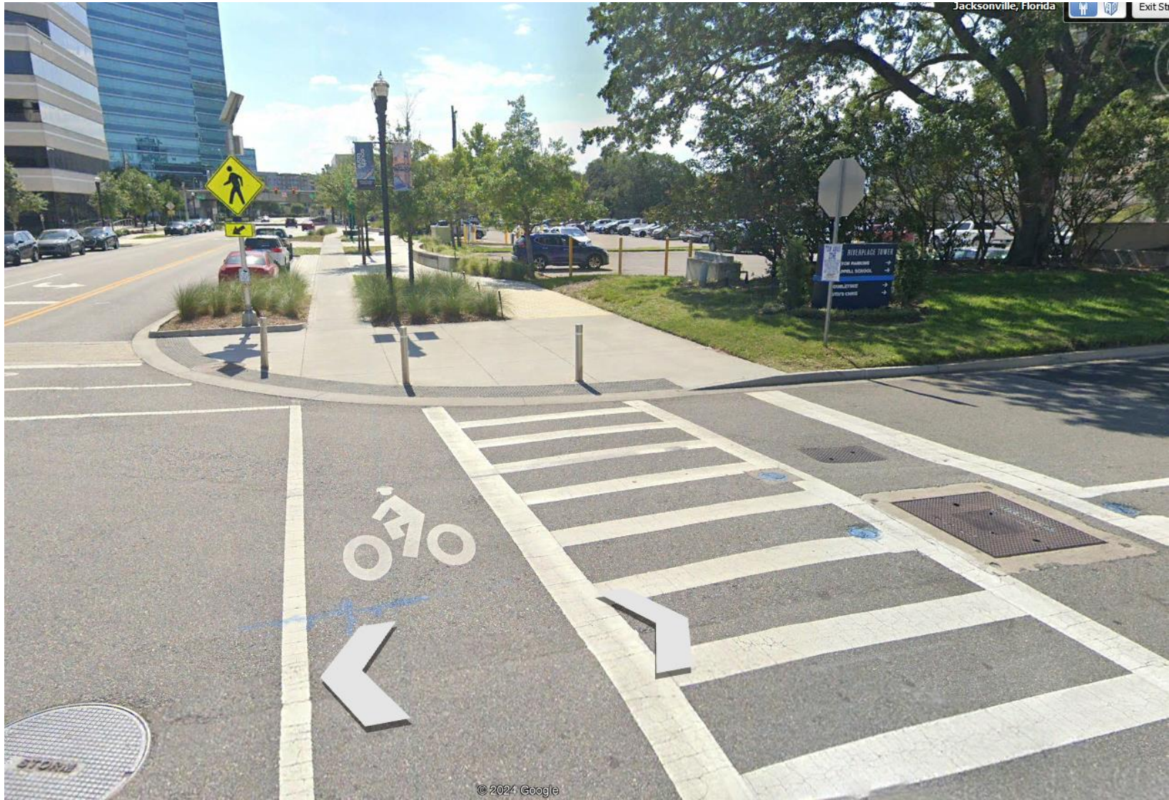
Existing facilities along Riverplace Blvd
