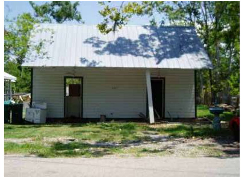
(a) Photo: Rubion Construction Co., LLC
