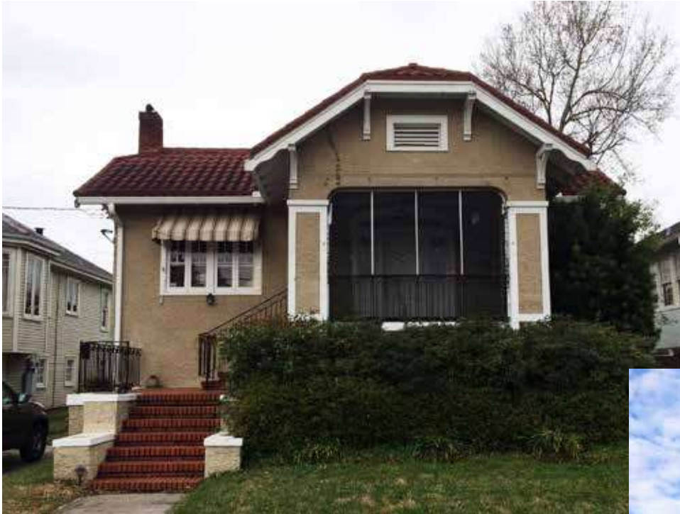
(a) Photo: Rubion Construction Co., LLC
