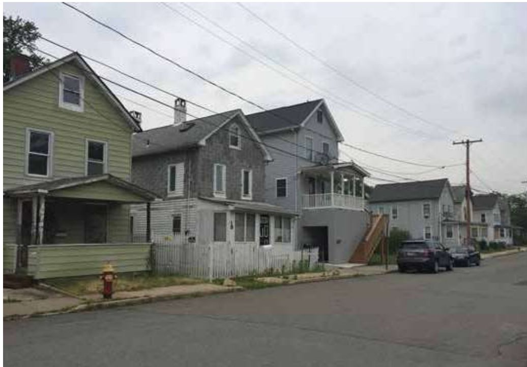
[99] Consideration should be given to the overall impact on the historic character and appearance of a district. A significantly different or random change in foundation height is inconsistent with the historic character of this district. Photo: Jennifer Parker/NPS
