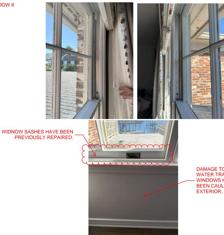
DAMAGE TO WALL BENEATH AND WATER TRAVELED TO LEVEL 1. WINDOWS HAVE TEMPORARILY **BEEN CAULKED FROM THE**
