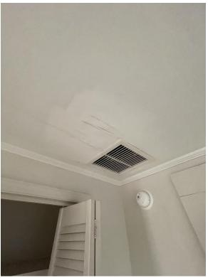
Photograph 8: Moisture Damaged Ceiling
