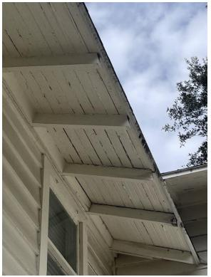
Photograph 6: Deteriorated Soffit Sheathing and Rafter Tails
