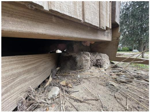
Photograph 2: Southwest Corner Settling with Cribbing
