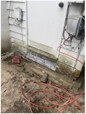
Photograph 4: Deteriorated North Wall Brick Foundation
