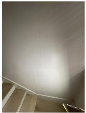
Photograph 7: Vertical and Horizontal Displacement of Interior Drywall
