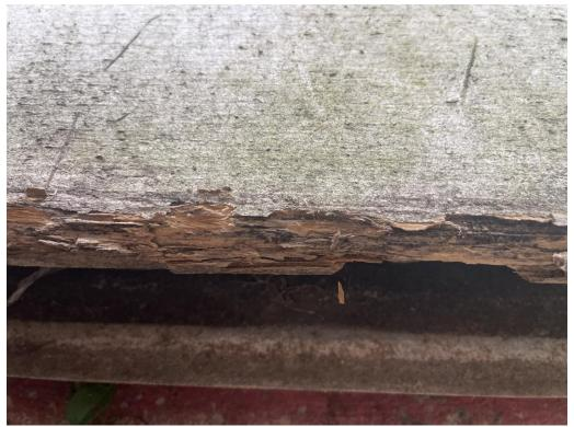
Photograph 5: Moisture and Termite Damaged Wood Siding
