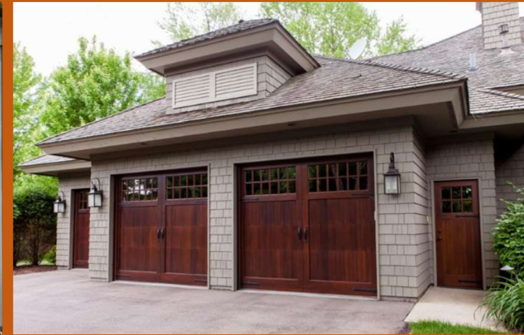
IN KEEPING WITH THE CHARACTER OF THE HOME, MATCHES THE PATTERN OF THE FRONT DOOR, AND THE BAYS ARE SEPARATED
