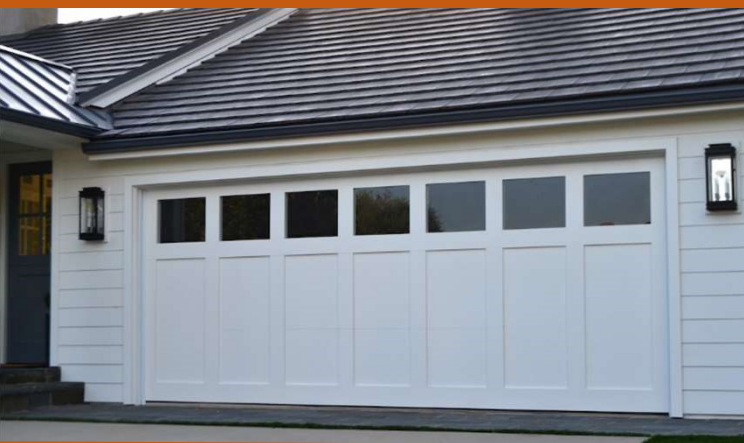
OVERSIZED GARAGE BAY OPENING
