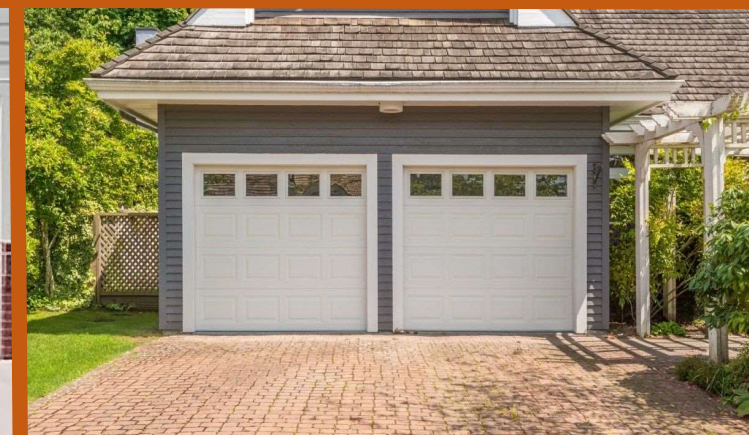
SIMPLE GARAGE DOOR DESIGN WITH SQUARE OPENINGS AND SQUARE WINDOWS WITH NO GRIDS
