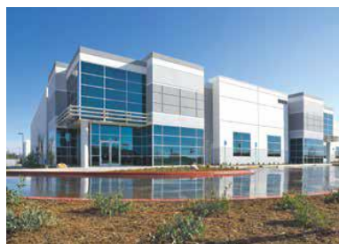
Southern California Logistics Center Victorville, CA
