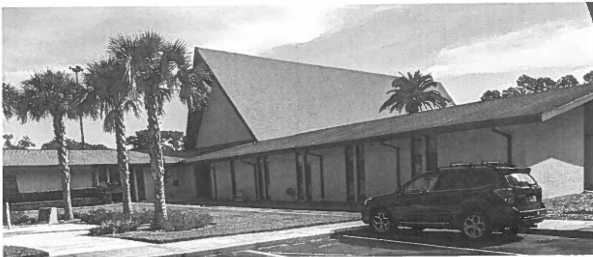
Bldg. 800 - 14,744 SF POW MIA Memorial Building Constructed in 1965
