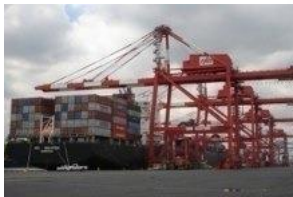
Newark Container Terminal
