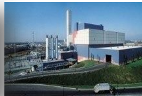
American Ref-Fuel Plant
