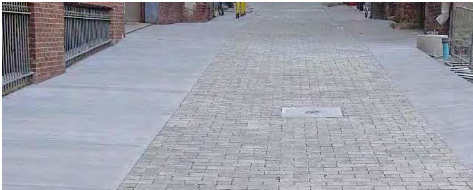
Figure 3. PICP used to reduce combined sewer overflows in Richmond, VA.
