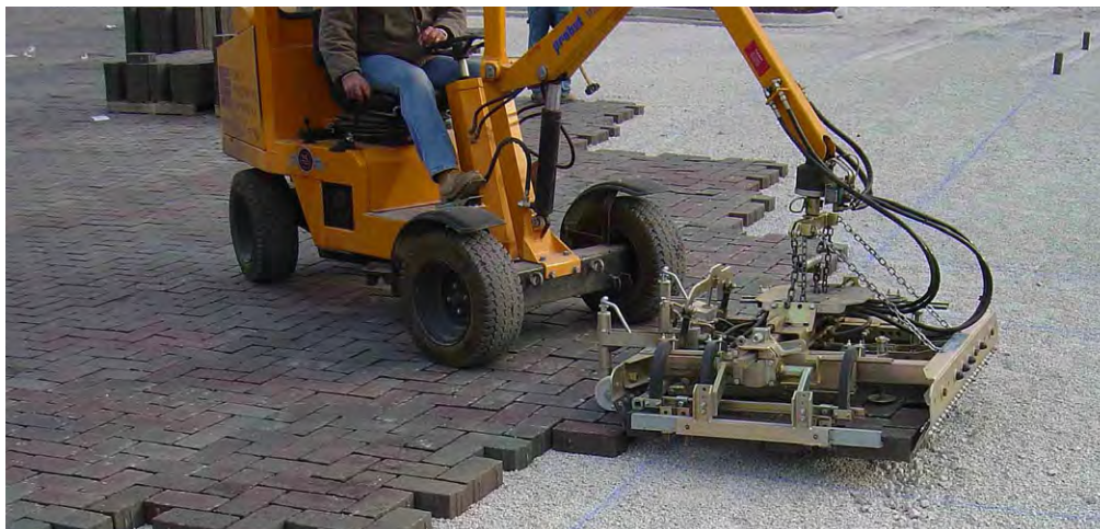
Figure 5. Mechanical installation of concrete paving units for PICP.
