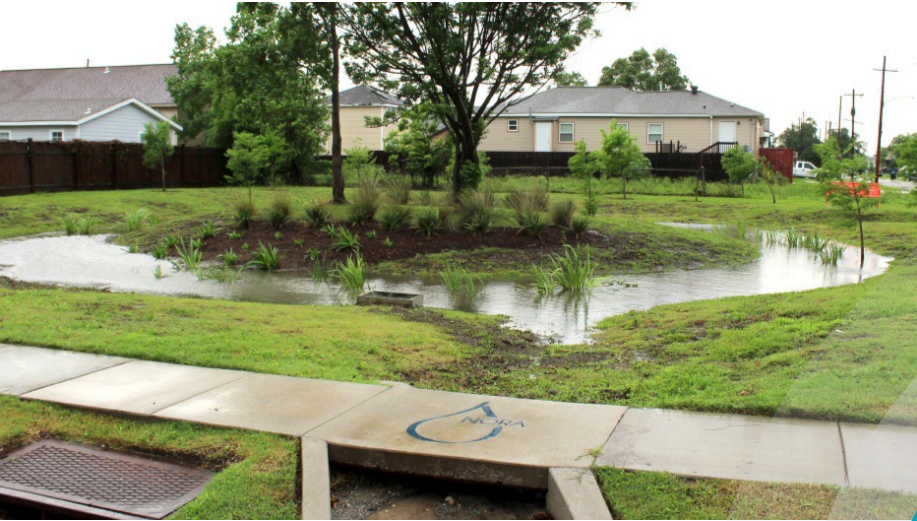
Reduced risk of flooding & damage
