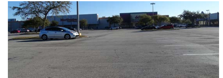
Excess impervious areas cause hot temperatures and runoff. Some older paved areas predate regulations requiring stormwater management.
