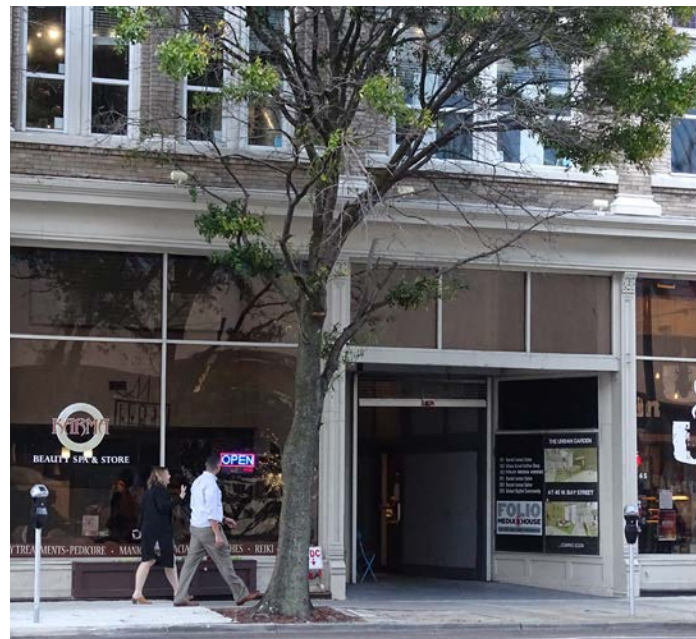
This downtown tree does not have enough room underground to support its roots and the tree is not healthy. The city can invest in better tree wells to ensure long term survival.
