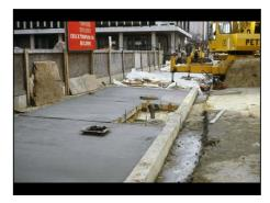
That little box on the sidewalk is my tree watering box. It connects to pipes under the sidewalk that are empty perforated lines. I can put water, liquid fertilizers, or compost heap in that box and energize the soil. We fill the trench up with soil and it is compacted lightly and we use the soil as the form for the bottom of the concrete.
