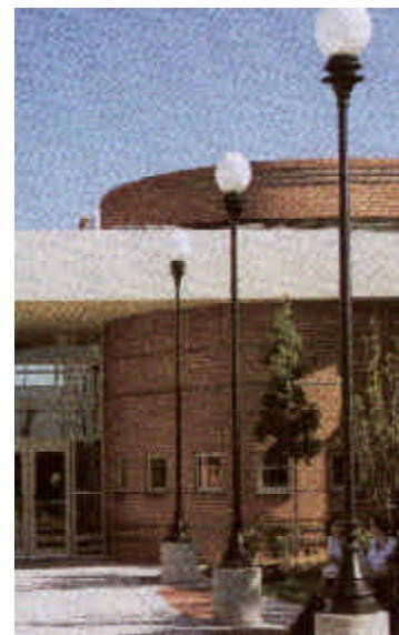
Art Deco style pedestrian light fixture
