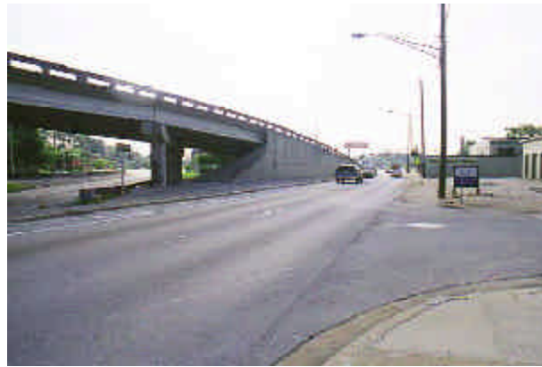
Overpass wall existing conditions
