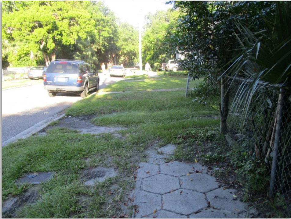
Figure 7: Sidewalk with overgrown vegetation, with potential sidewalk gap
