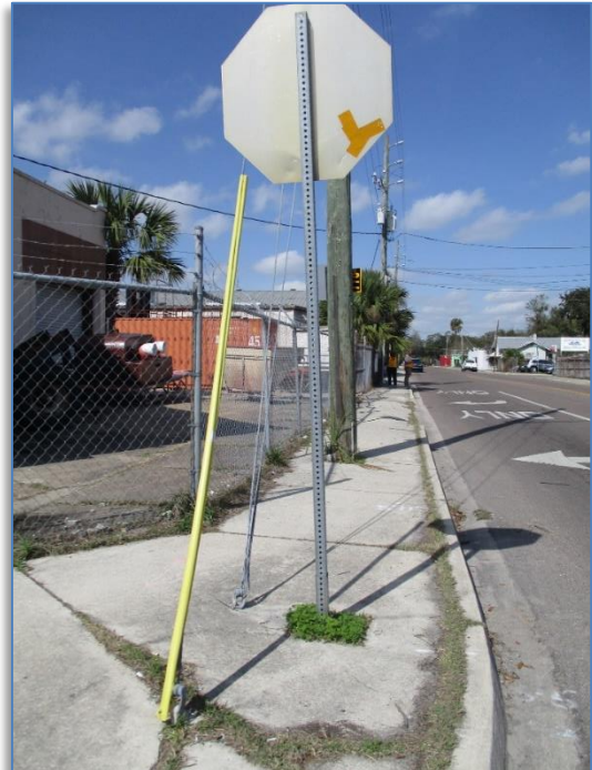
Figure 4: Utility poles and signs block the sidewalk
