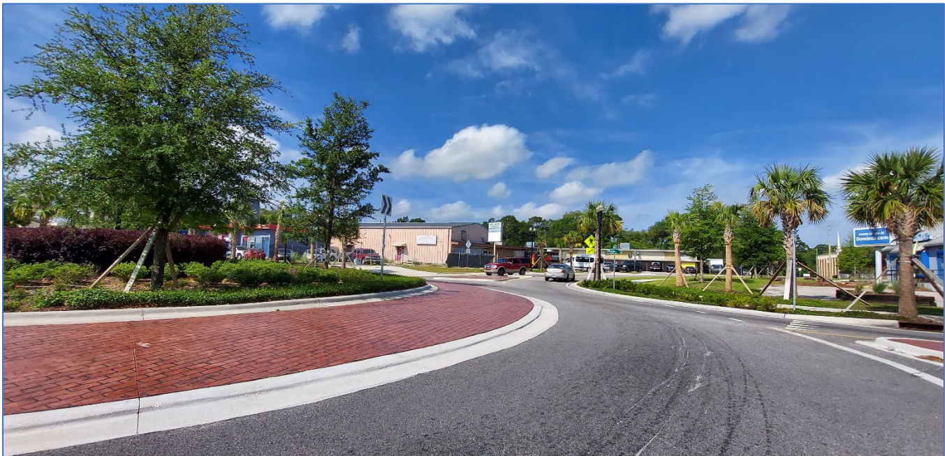
The intersection of Arlington Road and Rogero Road has been reconstructed into a roundabout. In the background, a vehicle is seen exiting onto Groveland Drive.
