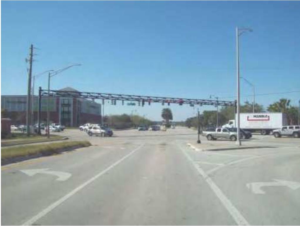
Looking west into the intersection along Tredinick Road
