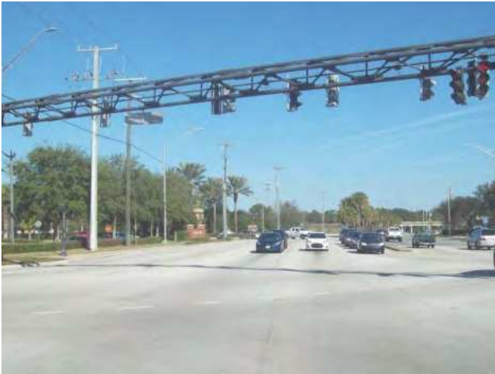
Looking north from the intersection along Monument Road
