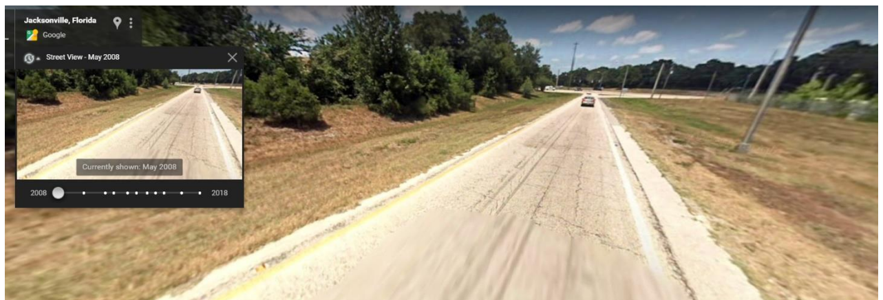
Figure 22 – 2008 Photo of Interstate-295 Northbound Off-Ramp
