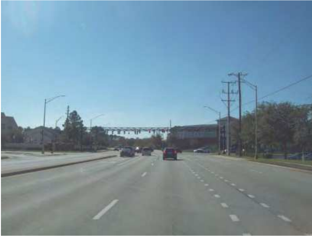
Looking south into the intersection along Monument Road
