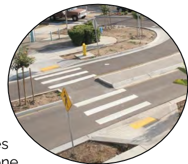
Pedestrian Refuge Island. Image Credit: FHWA
