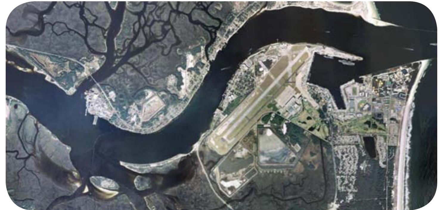
Aerial photo of the St. Johns River, Naval Station Mayport and Mayport Village (see Principle 4: Provide economic growth which advances neighborhood character, page 73)
