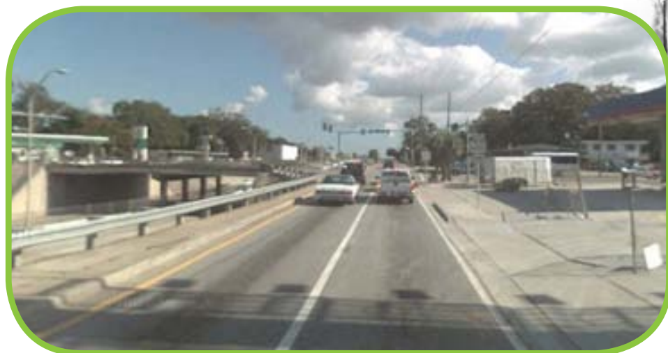
Photo: Existing conditions along the Arlington Expressway
