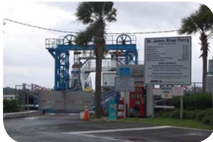
Photo: St. Johns River Ferry
