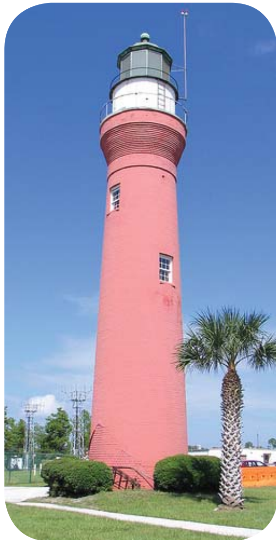
Photo: St. Johns Lighthouse
