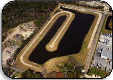
Cedar River Regional Stormwater Treatment Facility
