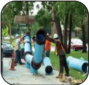
City of Jacksonville's septic tank phase-out program
