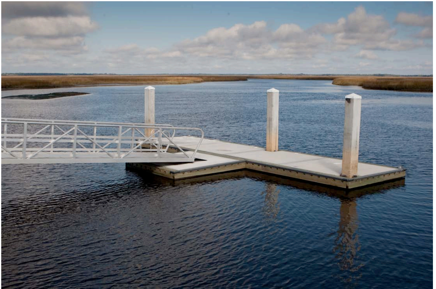
The gangway and floating dock at the Jim King Park and Boat Ramp at Sisters Creek Marina
