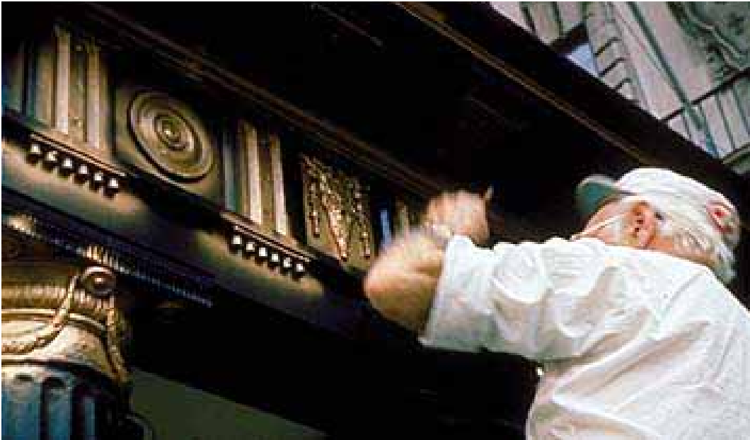
Repair of a decorative cornice. Preservation Trades Network Photo: Richard Wagner
