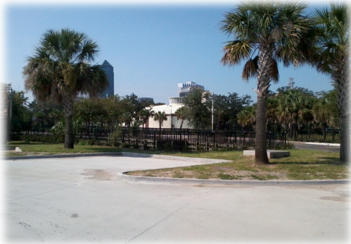
Main Street WTP
