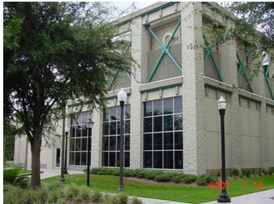
Hogan's Creek currently serves the Baseball Grounds and Arena, and has capacity to serve other customers, such as the EverBank Field, the Police Memorial Building and the Detention Center.
