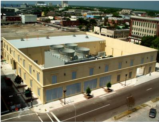
Downtown Facility serves the Library and Garage facilities, Jacksonville's new Courthouse, the JEA headquarters tower and other future downtown customers.
