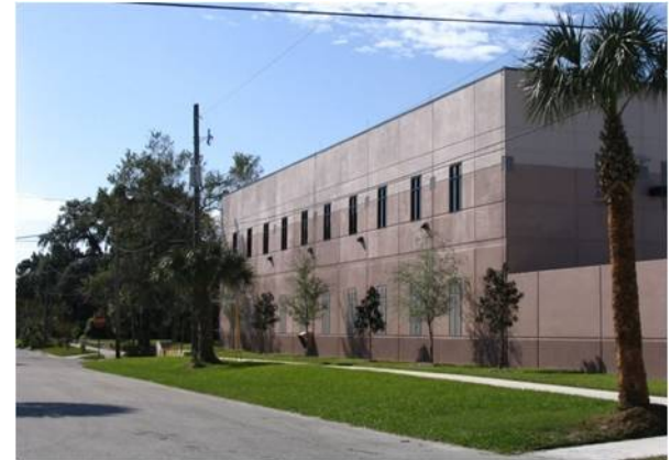
The Springfield Plant serves University of Florida's Proton Beam and Shands Healthcare, with a load capacity of 6,425 tons. The plant has expansion capability to over 10,000 tons.
