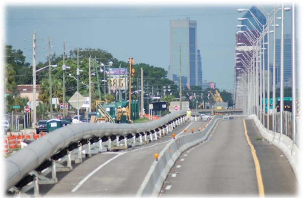
Water Transmission crossing the St. Johns River
